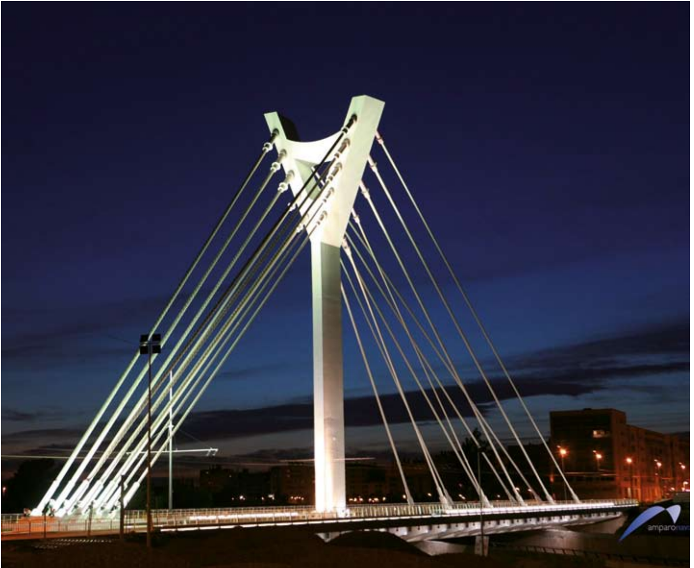
Castellón's TVRCas automated transport system crosses the Rio Seco via this new bridge
