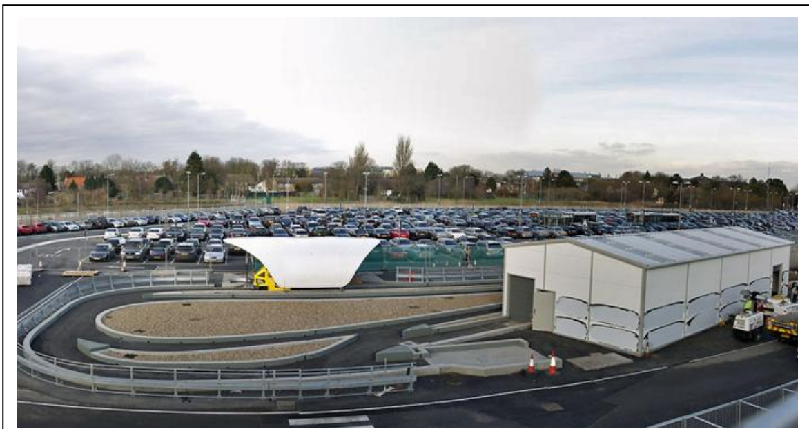
Figure 3 Station A and vehicle depot in Business Car Park
