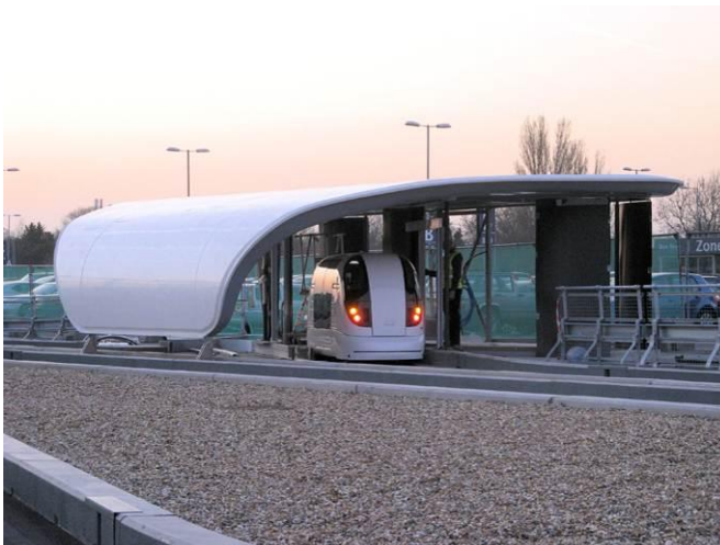
Figure 5.4 Heathrow car park station
