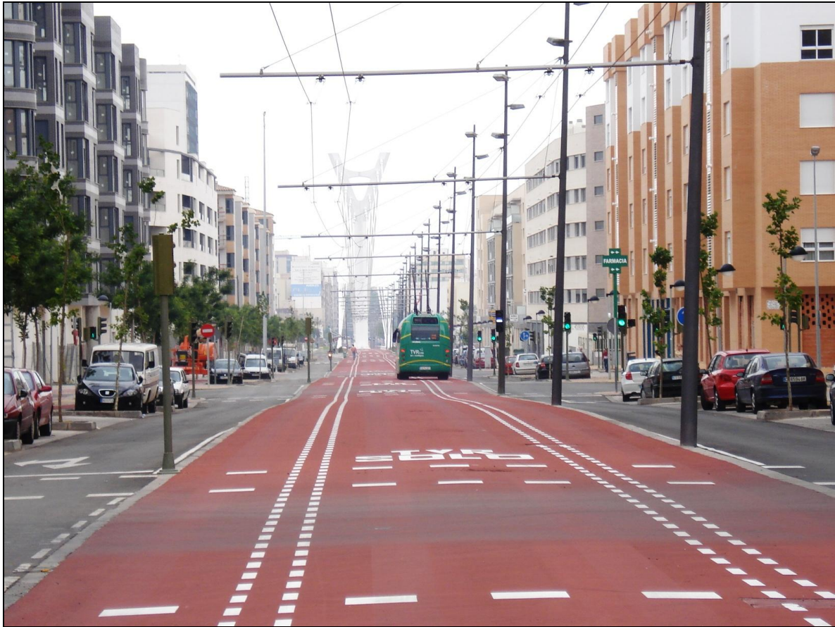
Fig.2 Example of a stretch of the dedicated lane segregated from the normal traffic
