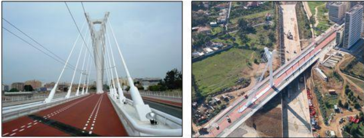
Fig.7 “Riu Sec” Bridge in Castellón Demonstrator
