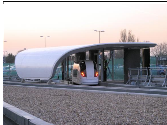
Figure 7: Station in car park
